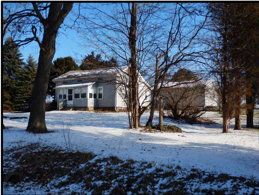
Figure 20. Northeast view TRU0104122 and its associated English barn from Tod Avenue SW (SR 45).
