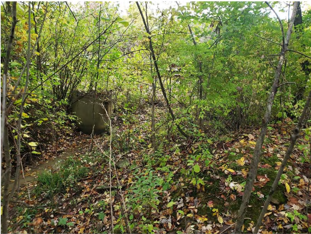
Photo 6: View of Stream 1 as it leaves the Site. Train tracks in distance. (Photo taken 10/16/2019)
