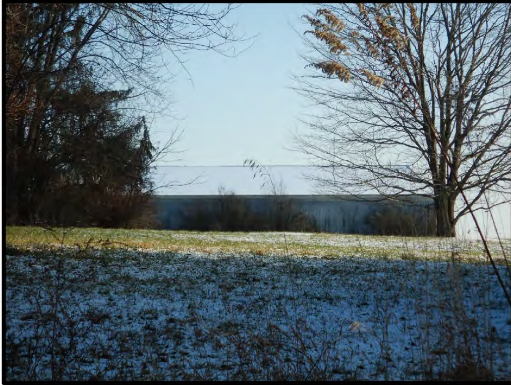
Figure 19. East view of a pole barn associated with TRU0104022 from Tod Avenue SW (SR 45).
