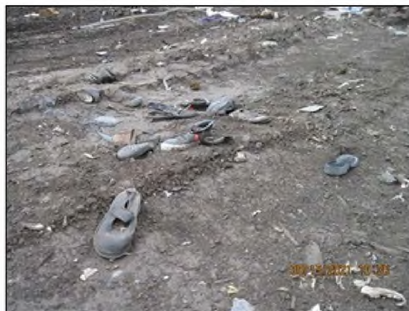
Fig 7 (Left) Area to the east of the working face that had inadequate cover and both MSW and C&DD were exposed.
