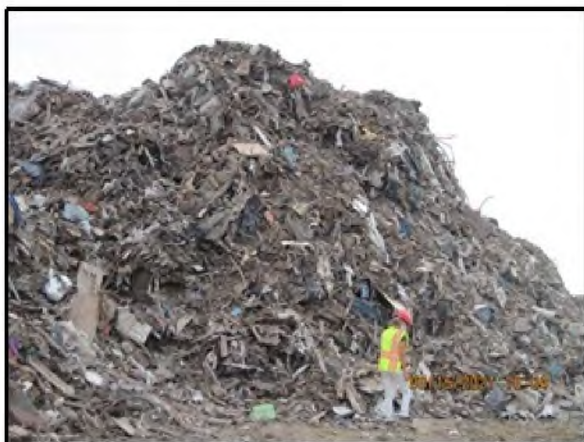
Fig 10 (Right): Area to the east of the working face that had inadequate cover and both MSW and C&DD were exposed.
