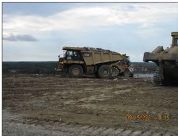
Fig 1 (Left): Unloading zone. The incoming loads of material were not deposited at a designated unloading zone and waste was pushed further into the working face.
