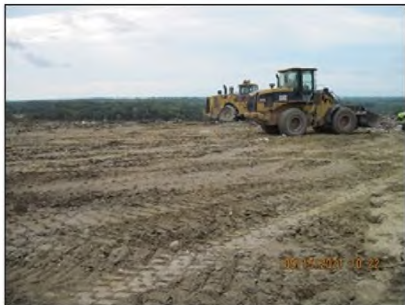
Fig 1 (Left): Unloading zone. The incoming loads of material were not deposited at a designated unloading zone and waste was pushed further into the working face.
