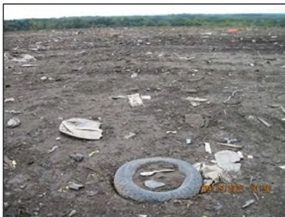
Fig 9 (Left): Area to the east of the working face that had inadequate cover and both MSW and C&DD were exposed.
