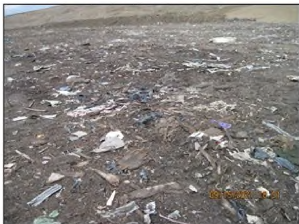
Fig 9 (Left): Area to the east of the working face that had inadequate cover and both MSW and C&DD were exposed.
