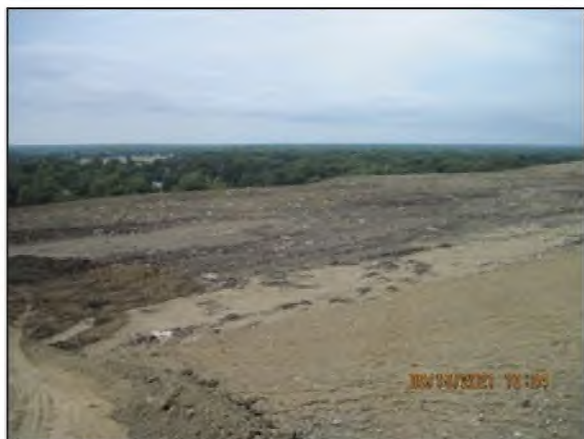
Fig 7 (Left) Area to the east of the working face that had inadequate cover and both MSW and C&DD were exposed.
