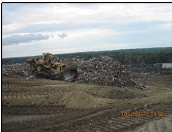
Fig 10 (Right): Area to the east of the working face that had inadequate cover and both MSW and C&DD were exposed.
