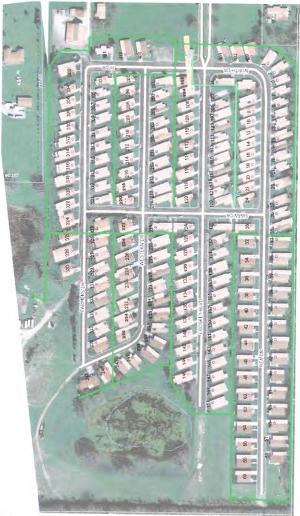
Country Haven Mobile Home Park PWS: OH 1201412 3-7-2017 * Light green water line is galvanized water line, but dark green is PVC water lines. " NO LEAD SERVICE LINES" The Park was built around 1981. Galvanized water service lines were replaced with PVC in the late 70's and finished in the late 80's. Most of the mobile homes predate 1998 and have the potential to have lead solder and fixtures >8% lead and have a higher risk of contributing lead to the drinking water.
