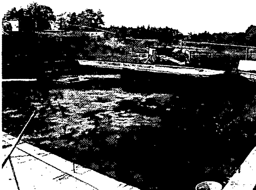
Figure 2: Surface of the north sand filter covered in thick black sludge.
