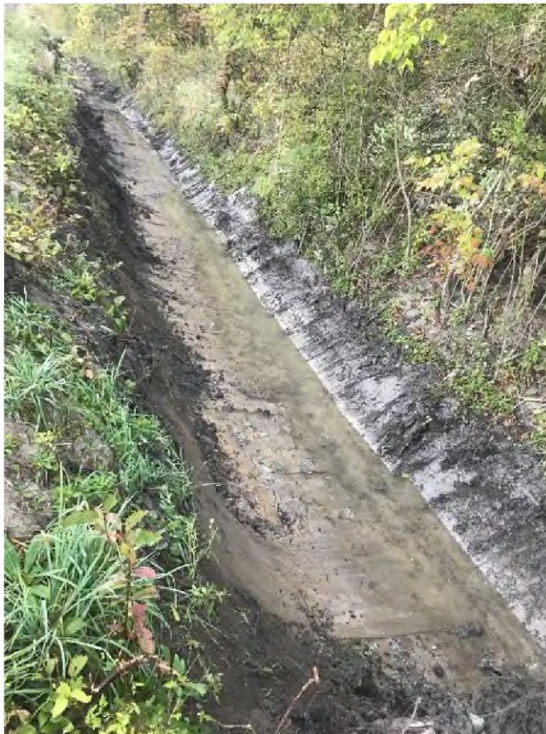
September 28, 2021 – Excavation of sediment and at least 6" underlying clays in Dawley Ditch. Looking North.
