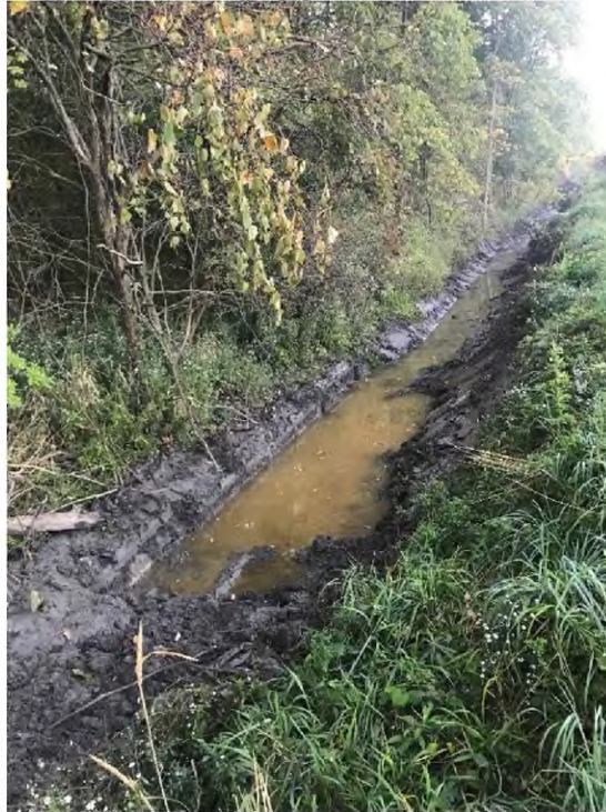
September 28, 2021 – Excavation of sediment and at least 6" underlying clays in Dawley Ditch. Looking North.
