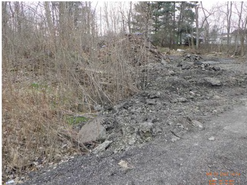
Figure 2. View of access drive showing recently introduced ground asphalt fill in a wetland, facing northwest.
