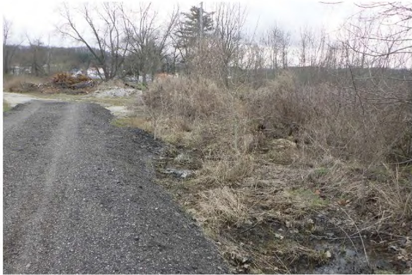
Figure 1. View of access drive showing recently introduced ground asphalt fill in a wetland, facing southeast.
