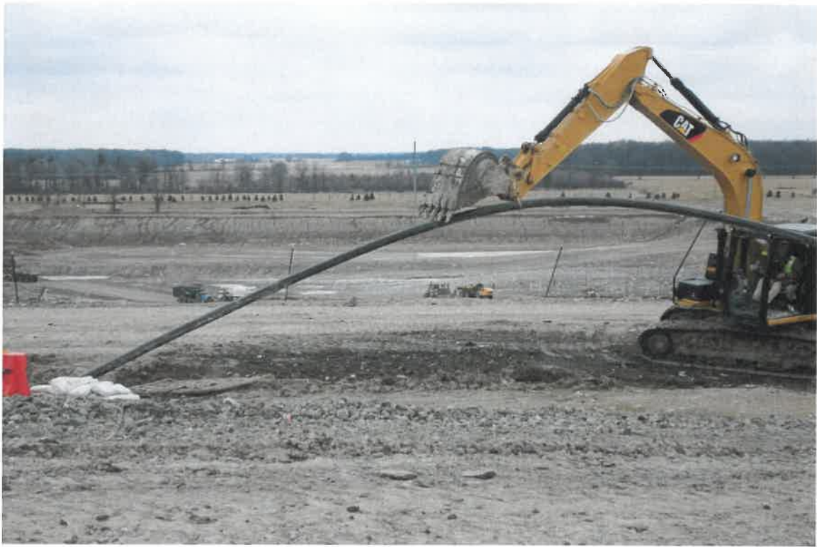
Photograph 15. Installation of 6" well casing in bore for redrill EW303R, facing north.
