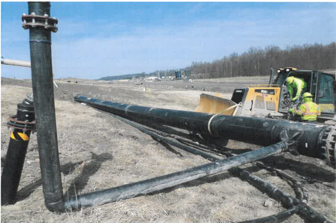
Photograph 34. 6" lateral fabrication for EW32R off of the 24" replacement header, facing northeast.
