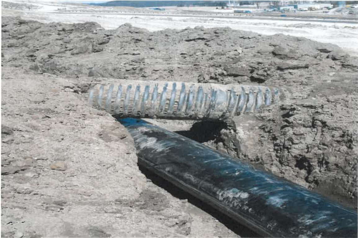
Photograph 29. 24" header repair on east side of landfill; 24" header was installed below the pre existing ADS drainage pipe, facing northeast.
