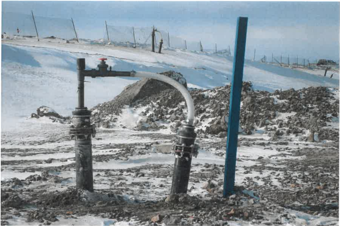
Photograph 19. Completed well EW303R with blue road crossing markers, facing southwest.
