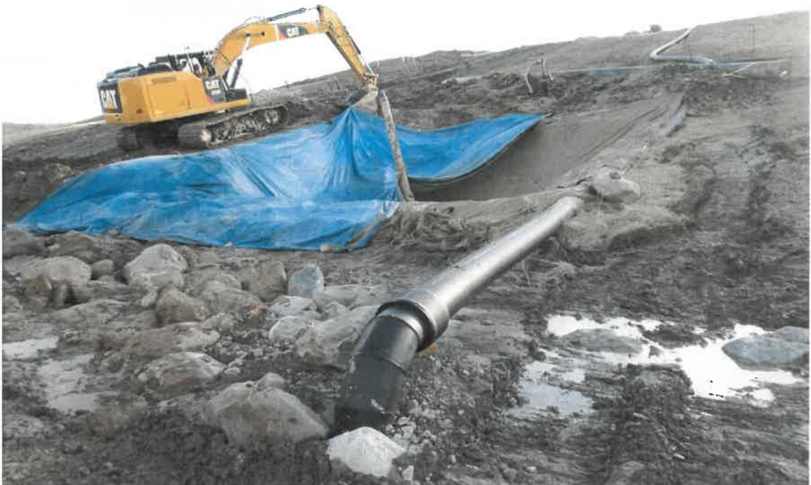
Photograph 30. Tarping the 24" header tie in point to prevent odor and liquid infiltration, facing southwest.
