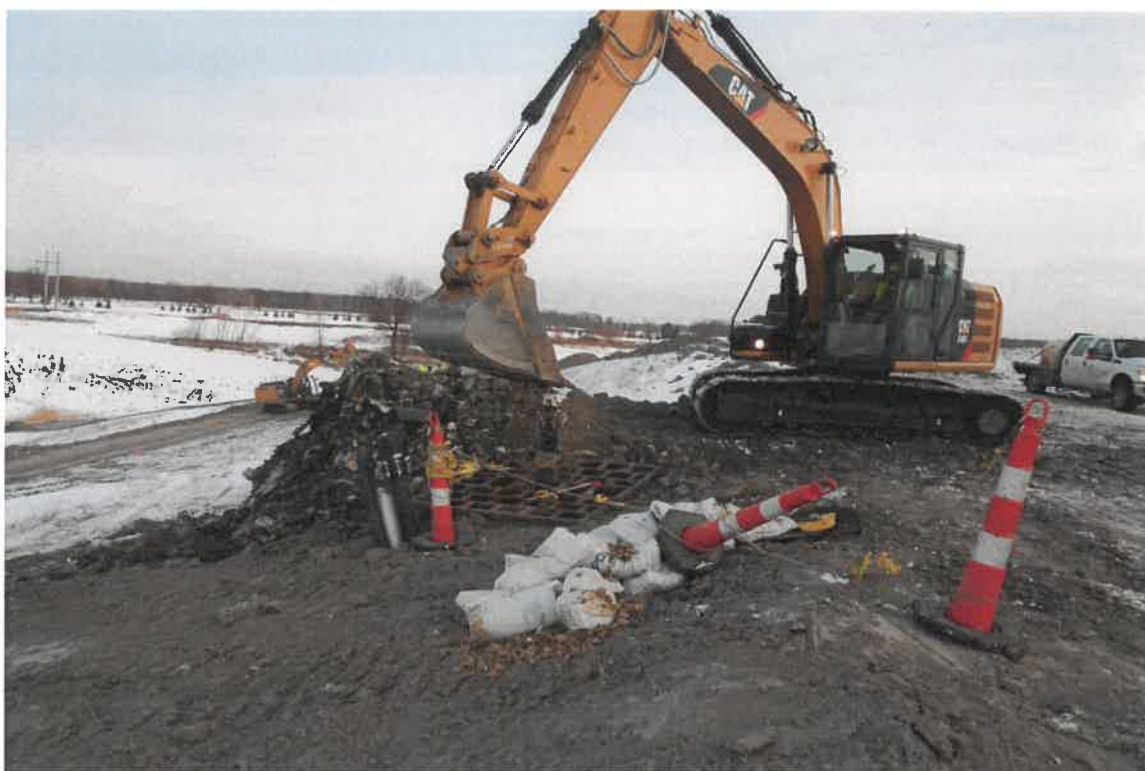
Photograph 13. Number 4 stone installation for new well EW329, facing northeast.
