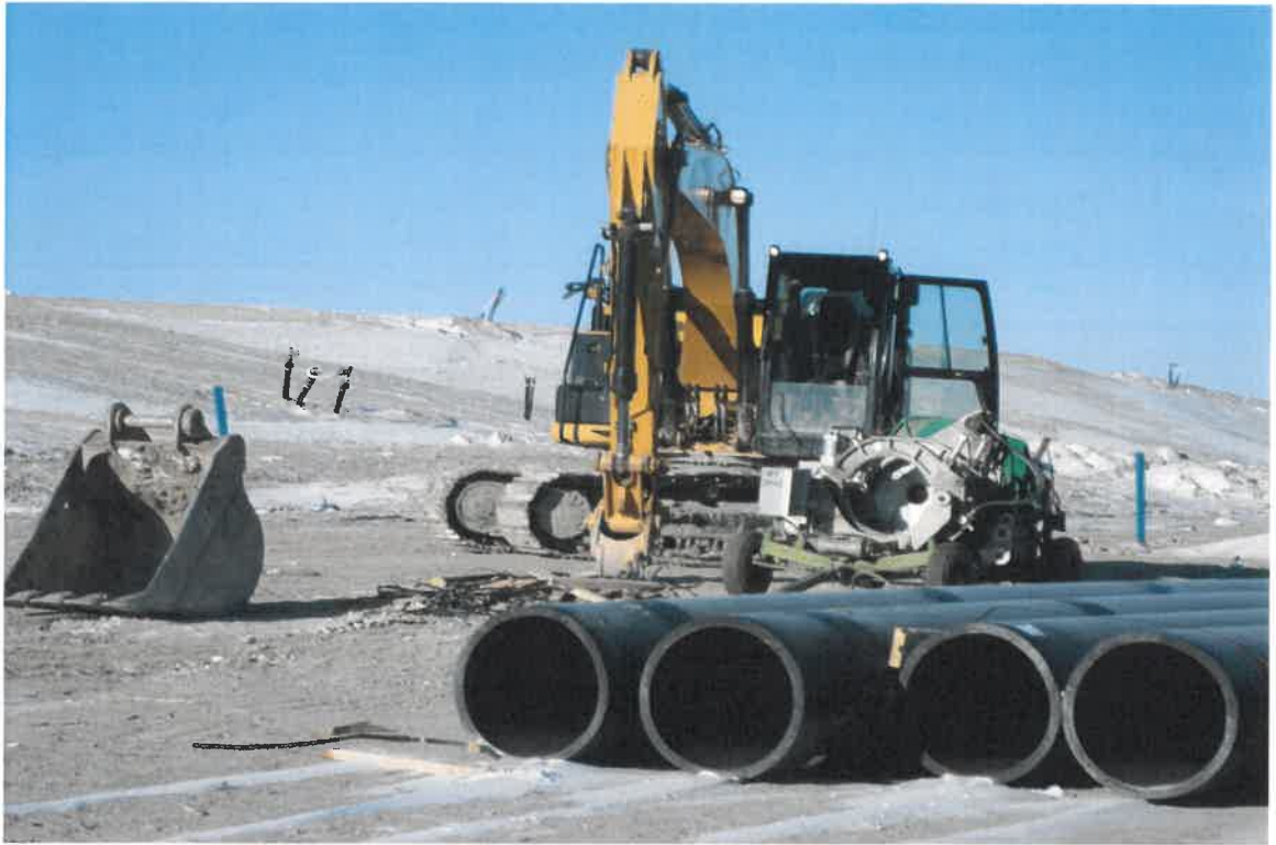
Photograph 27. Supplies for 24" header line replacement to repair 24" vacuum loss, facing southwest.
