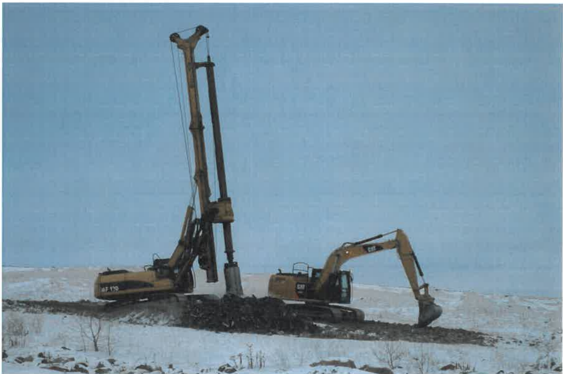
Photograph 28. Drilling EW173 and cleaning up of drill cuttings for transfer and disposal in the active phase, facing southwest.
