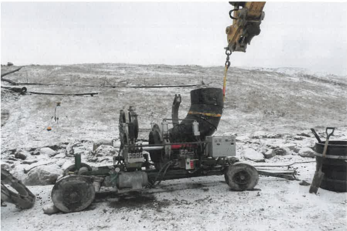
Photograph 32. Fusion of 24" tie in piece; pictured is SDR17, 24", 90° adapter, facing southwest.
