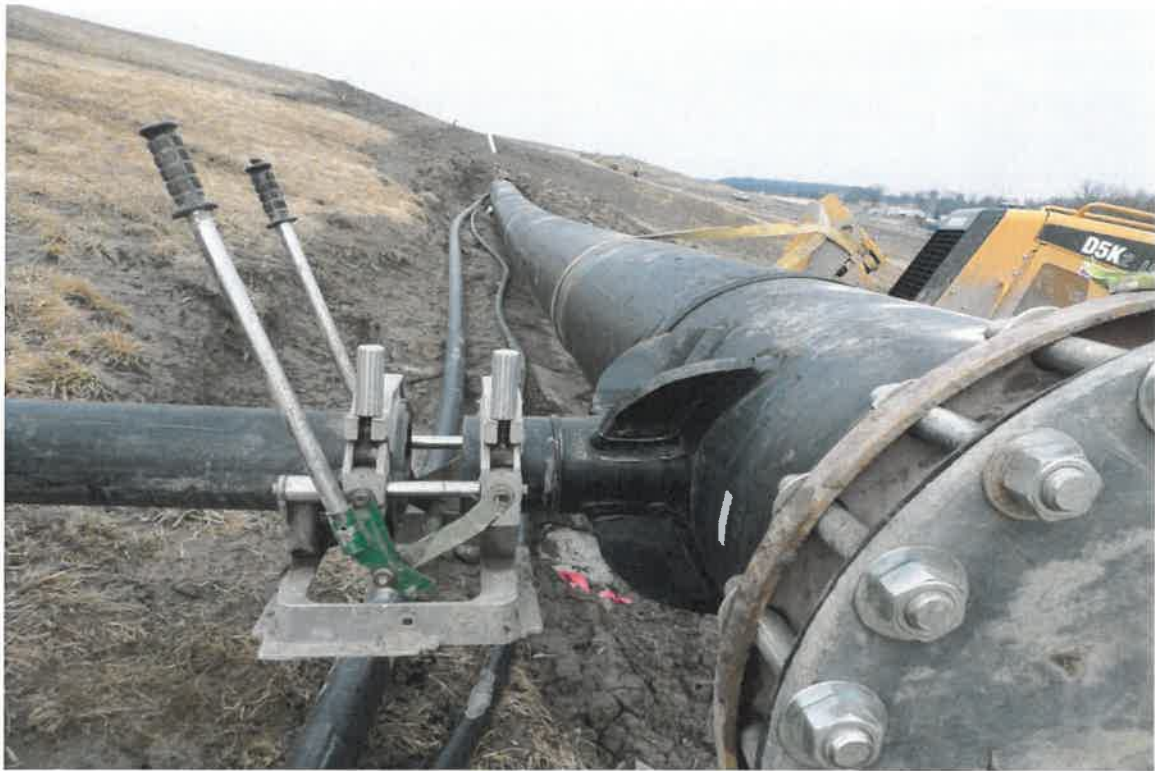
Photograph 33. Fusion of 6" lateral to 24" header at the 6" gusseted branch saddle for EW32R; shows flange connection to pre existing 24" header, facing north.
