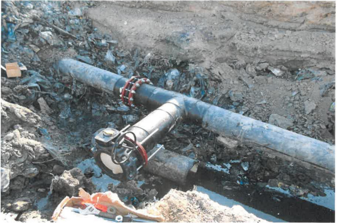
Photograph 5. New 12" header isolation valve near EW55R, facing southeast.
