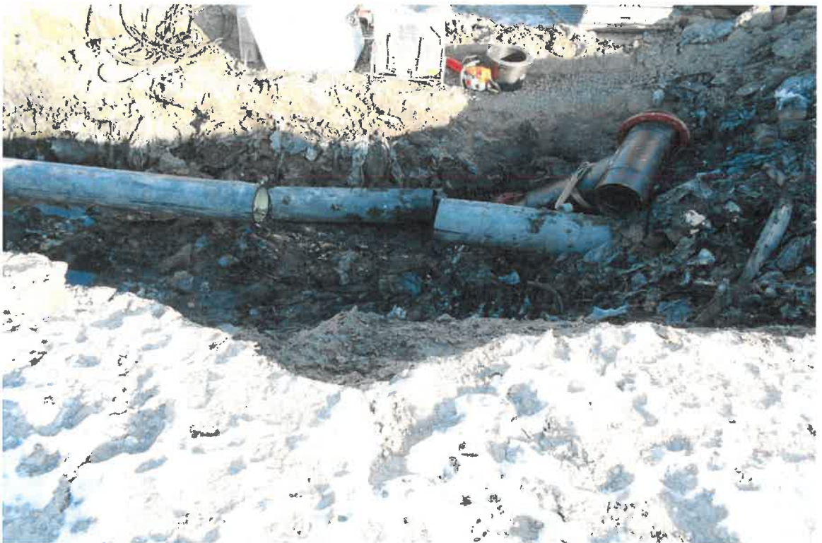
Photograph 4. 12" header cut for placement of 12" T and isolation valve.
