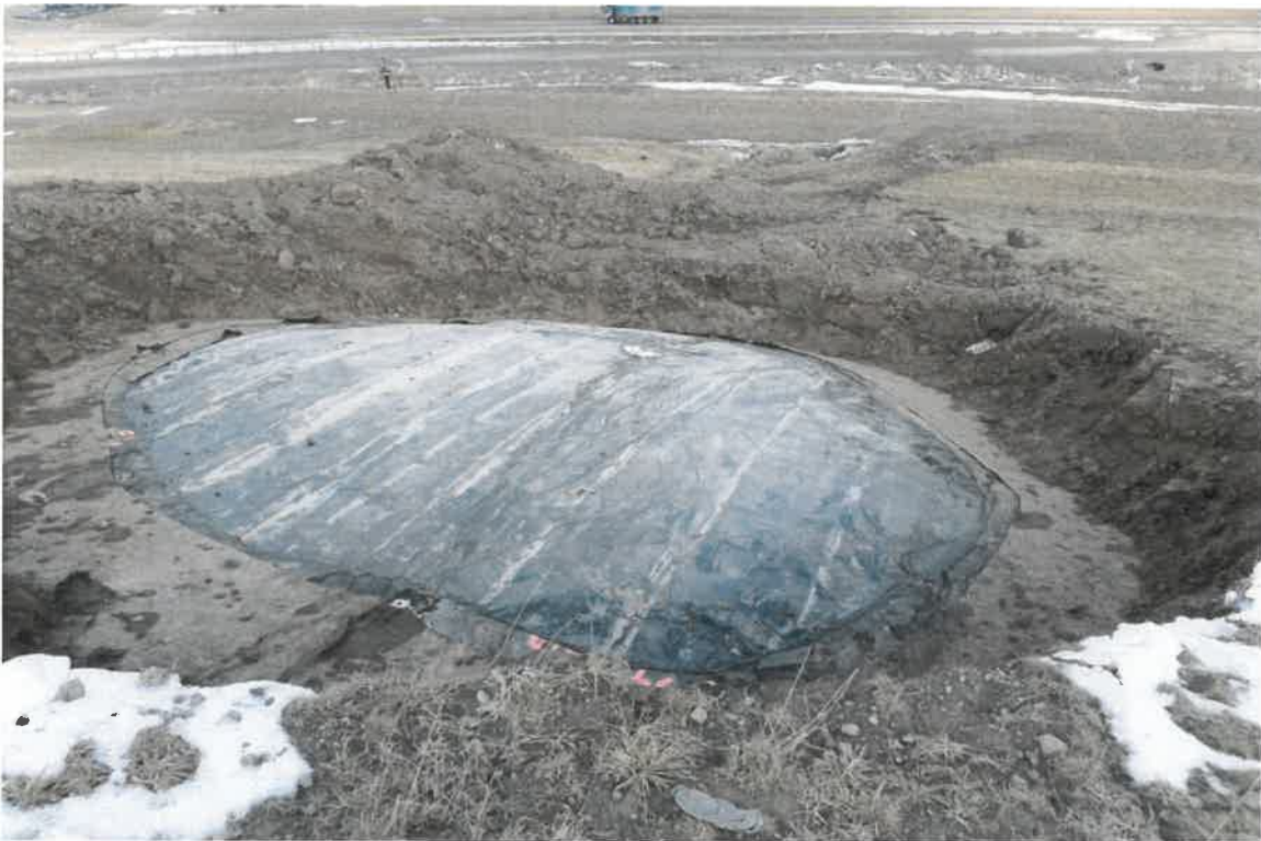
Photograph 26. Liner repair of east slope trouble shooting area; header was too deep to be excavated in this area; opted to replace entire 24" header on east slope.
