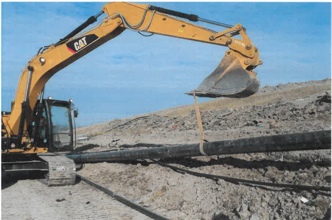
Photograph 10. 12" header being pulled into trench for placement.
