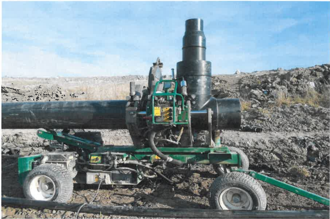
Photograph 9. 12" fusion machine; welding 12" T to 6" reducer, facing east.
