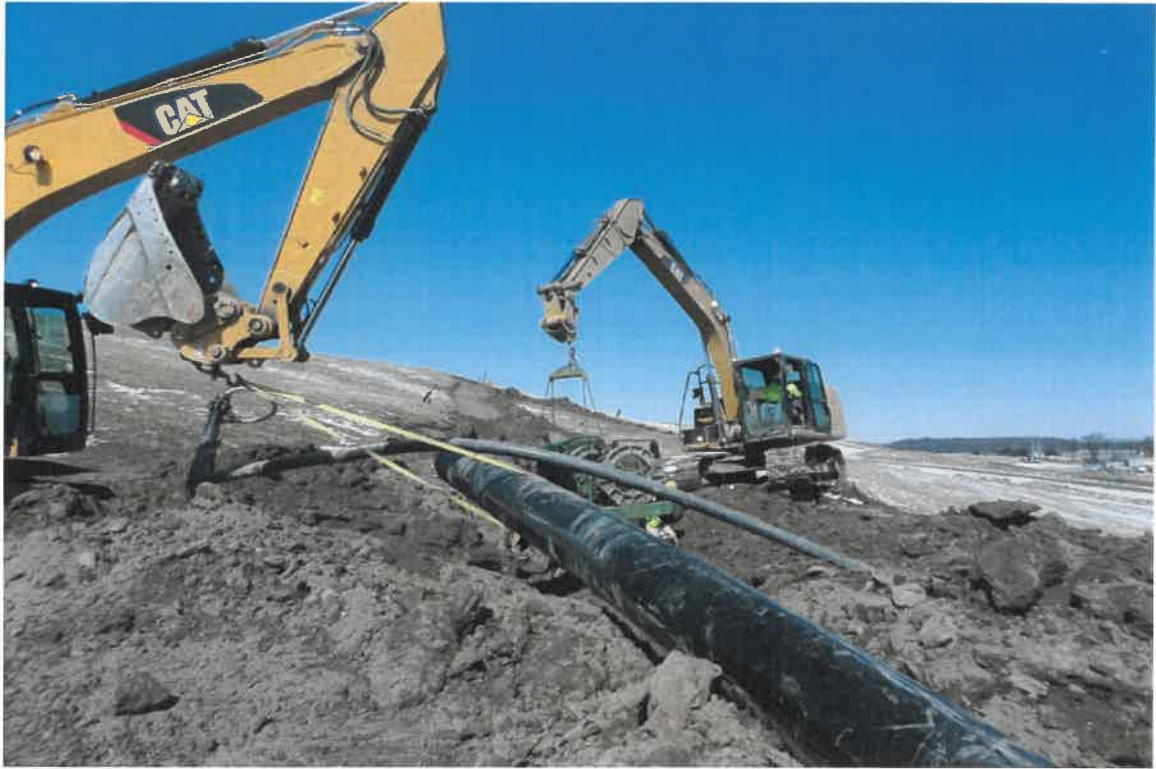
Photograph 31. Placement of 24" replacement header and 2" air line in the trench, facing north.
