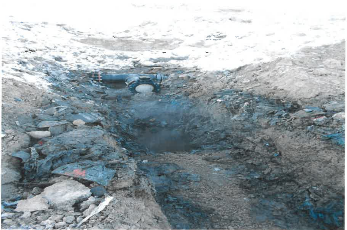
Photograph 7. Dug a rock sump for leachate drainage near the new 12" header isolation valve, facing south.
