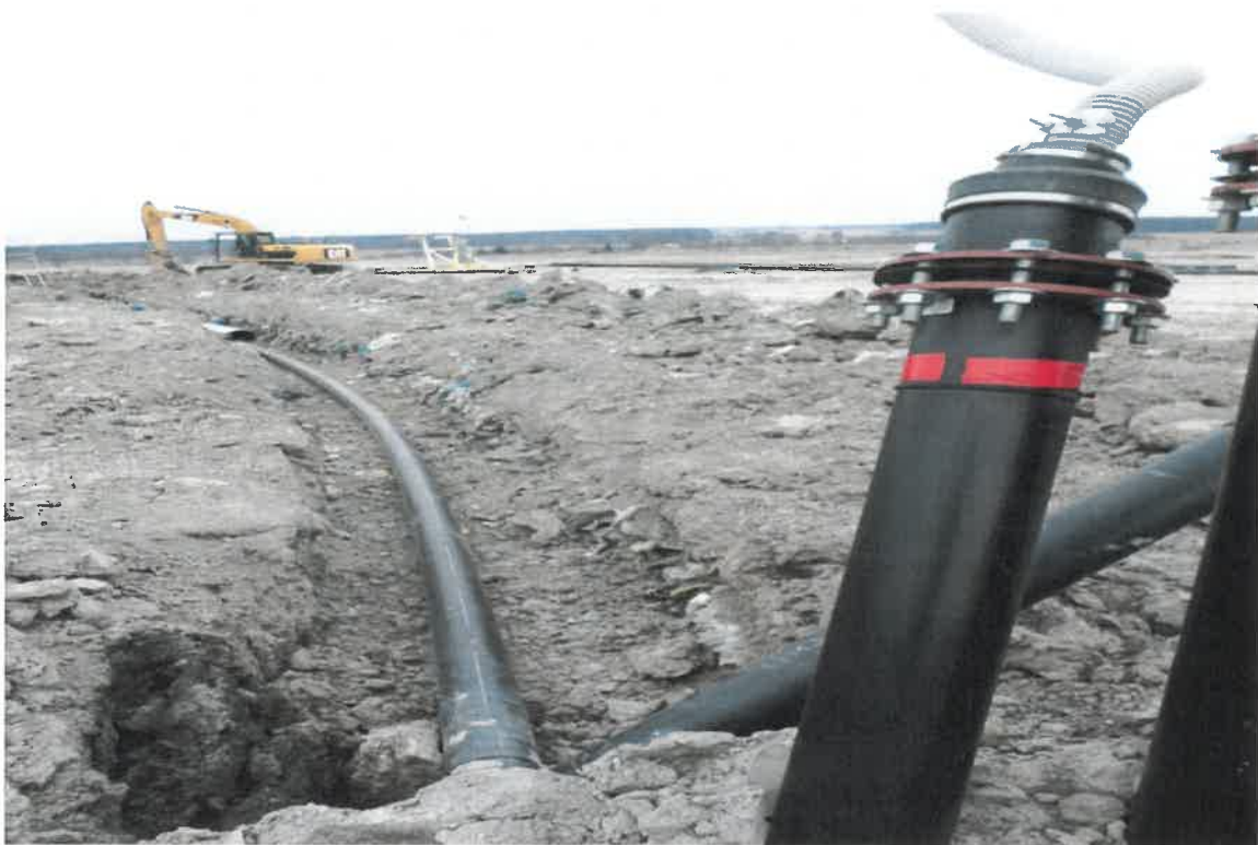
Photograph 16. 6" lateral installation and 12" CMP (corrugated metal pipe) road crossing at EW303R, facing north.
