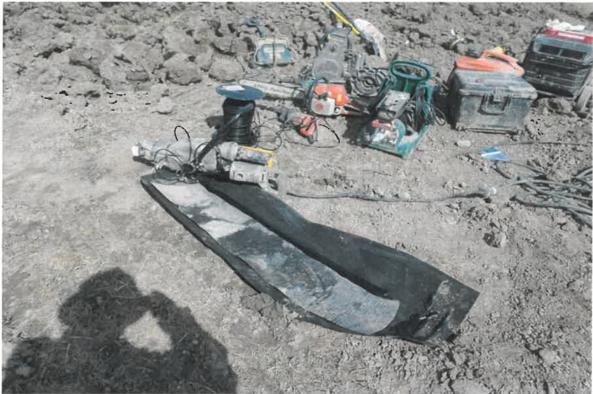
Photograph 35. Test panel to create test “bones” for the tensiometer prior to repair of the east side liner.
