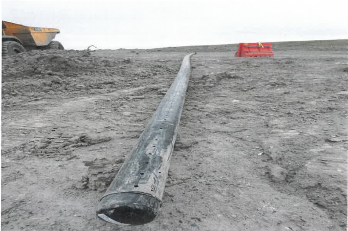
Photograph 17. Well casing prior to installation EW333; shows SDR17 6" perforated pipe, facing south.
