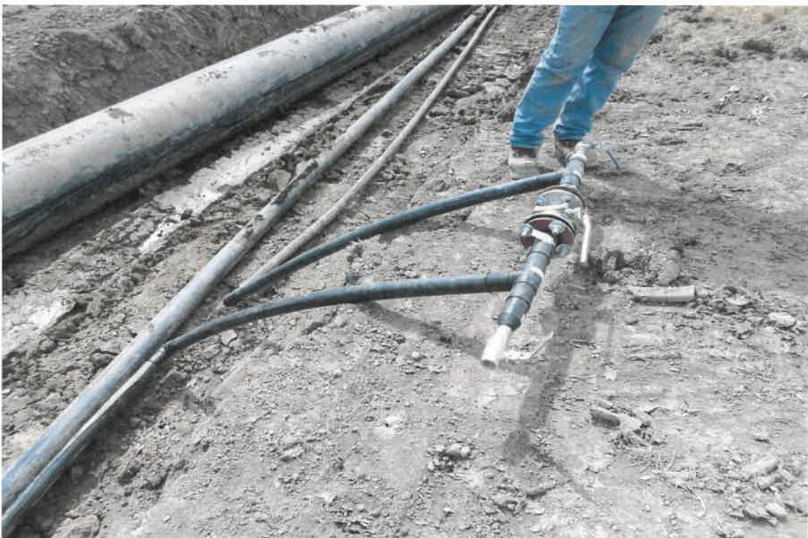
Photograph 36. F24" header replacement, 2" air line, and 2" x 4" dual contained force main including air isolation valve at EW31R.
