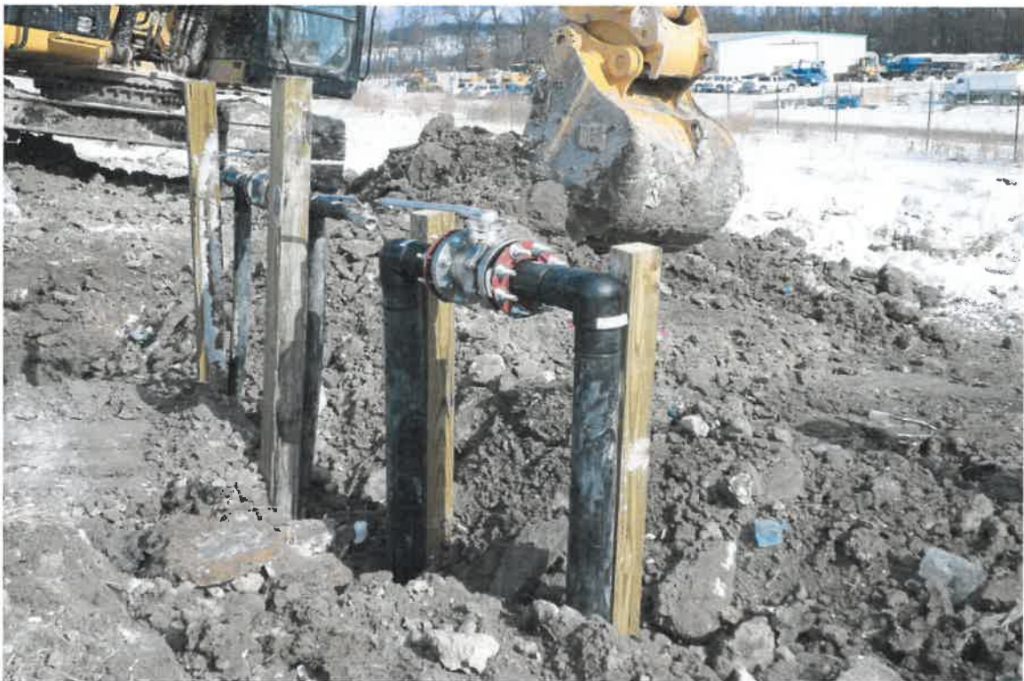
Photograph 24. Installed air and force main isolation valves on east side of GCCS system to trouble shoot potential system pressure loss, facing northeast.
