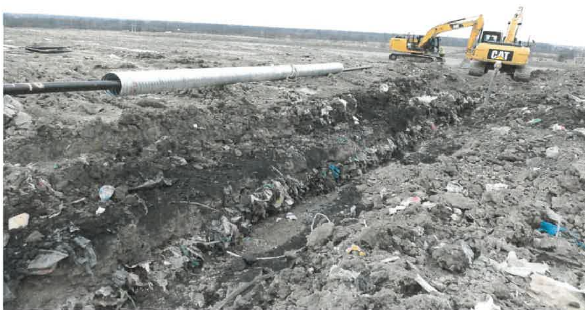
Photograph 14. 12" CMP (road crossing) for 6" remote lateral installation for EW45R3, facing north.
