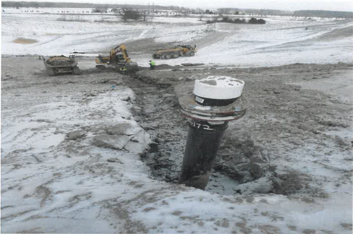
Photograph 23. Trenching 6" lateral from new well EW172 to obtain a vacuum source from EW327, facing northeast.
