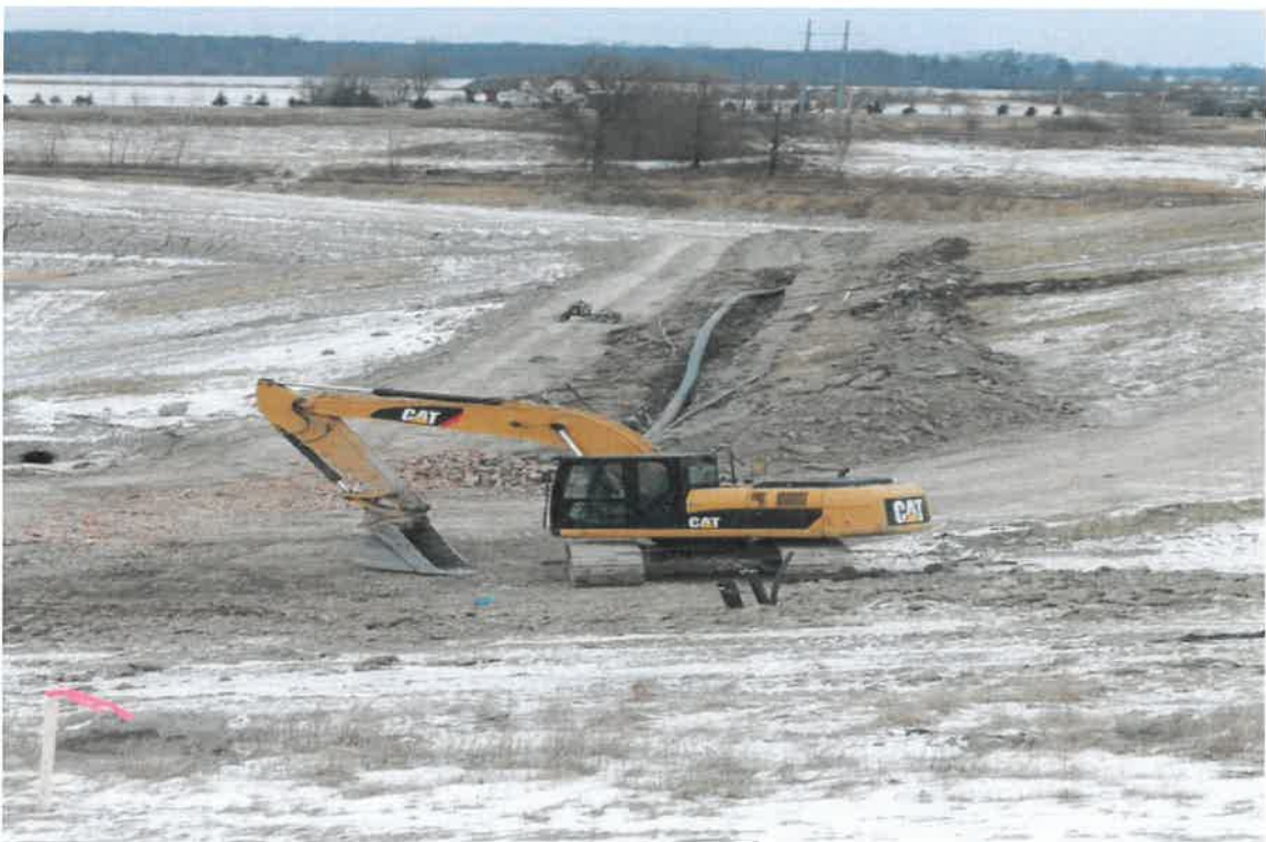
Photograph 2. 12" header installation with brick visible from road crossing (12" CMP) from 50R3 to 12" header, facing northeast.
