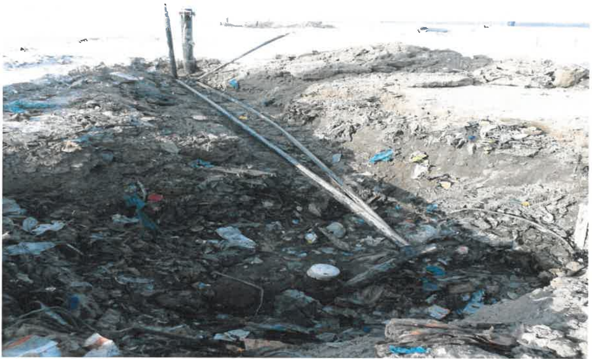
Photograph 21. Extension of air and force main from EW42R to EW42R2 and proper abandonment of EW42R, facing north.
