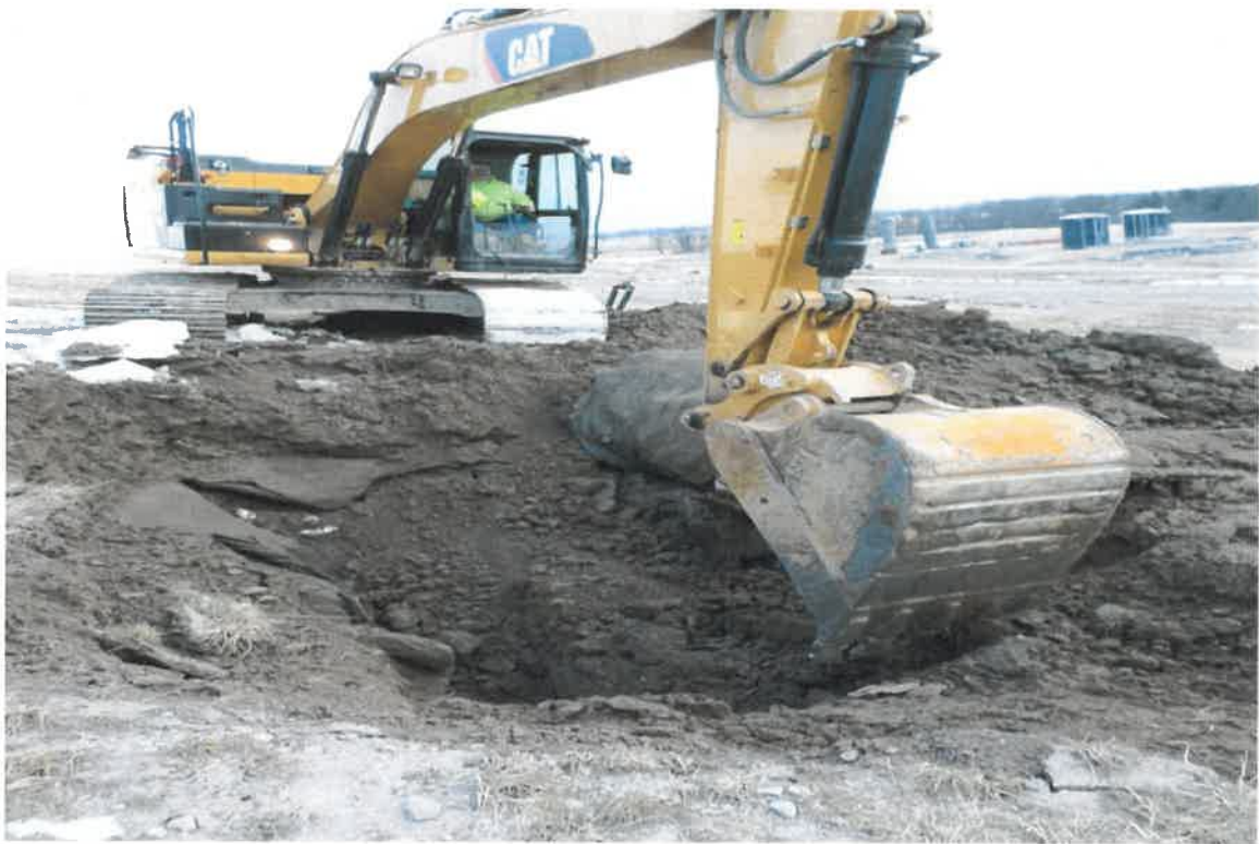
Photograph 25. Uncover east slope cap area to trouble shoot the source of a 20.0" w.c. (water column) vacuum loss at the request of SCS and the Site, facing north.
