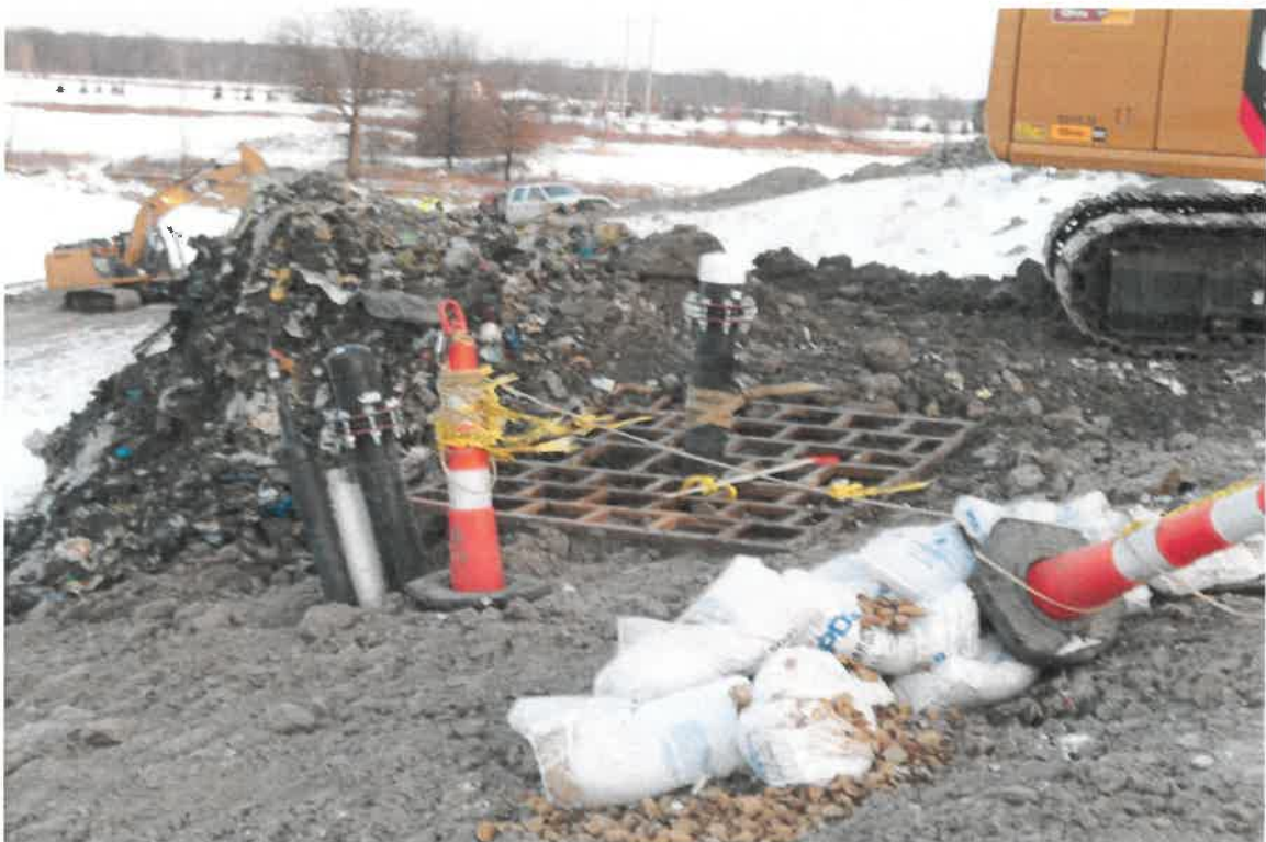
Photograph 12. Set casing on new well EW328, facing northeast.
