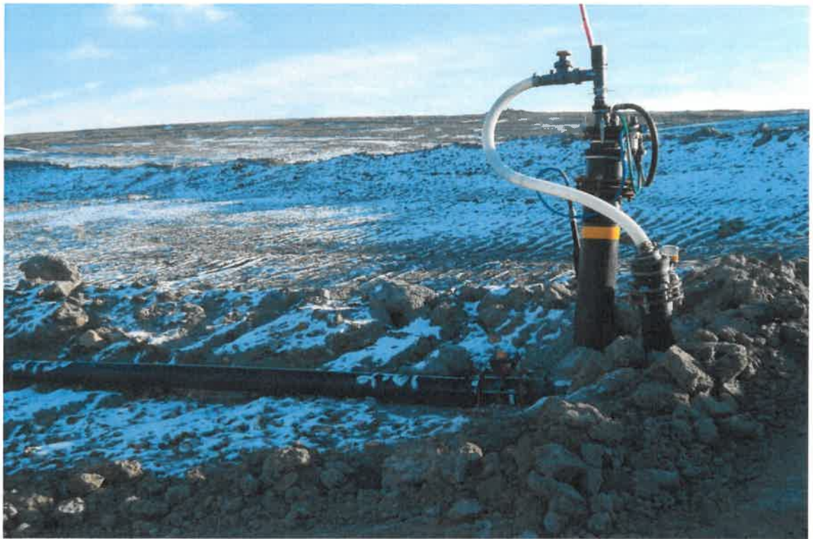
Photograph 3. EW54R2 prior to removal of 6" jumper lateral, facing east.
