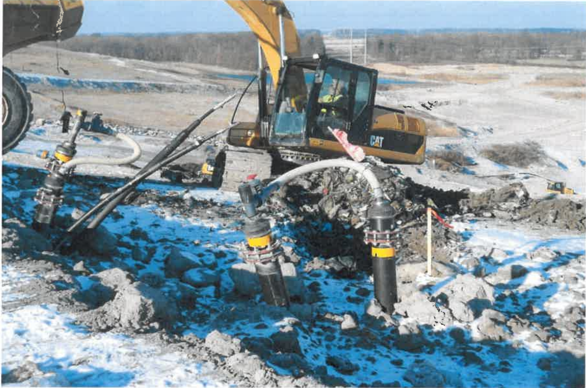
Photograph 1. Excavation of tie in point for 12" header on north slope, facing west.
