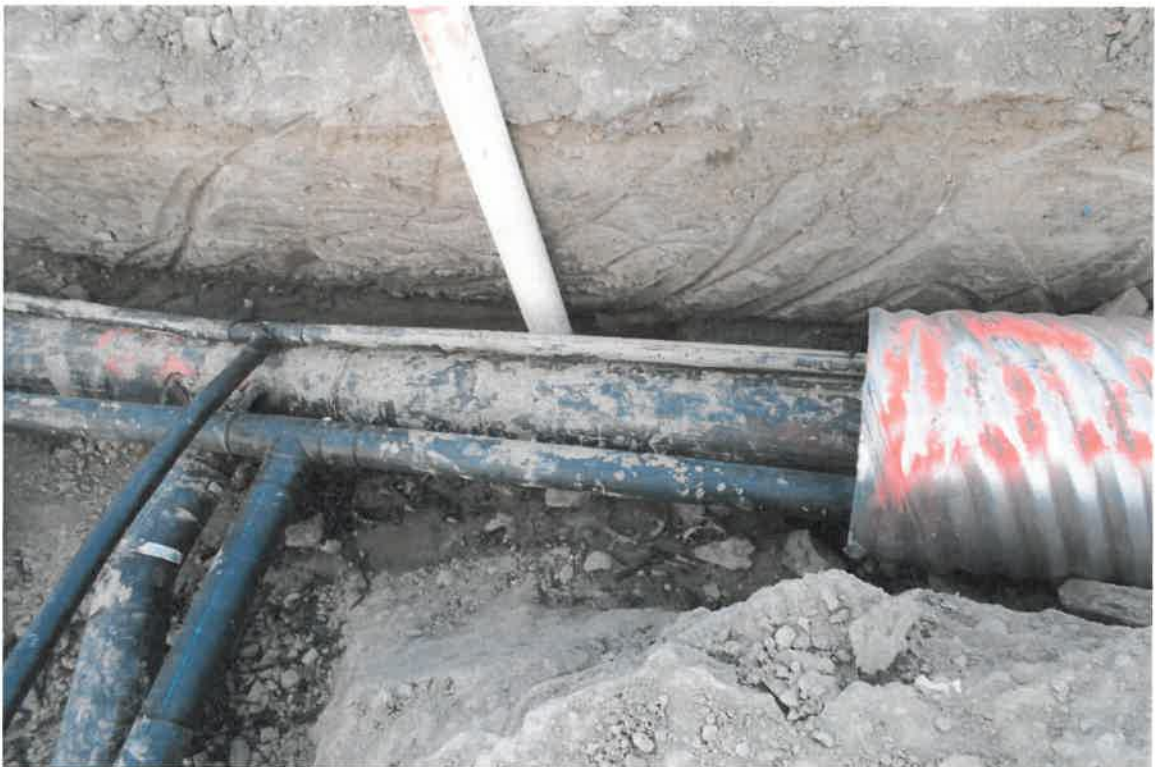
Photograph 8. 12" CMP road crossing; 6" lateral, 2" air, and 4" force main for future tie in to EW327.
