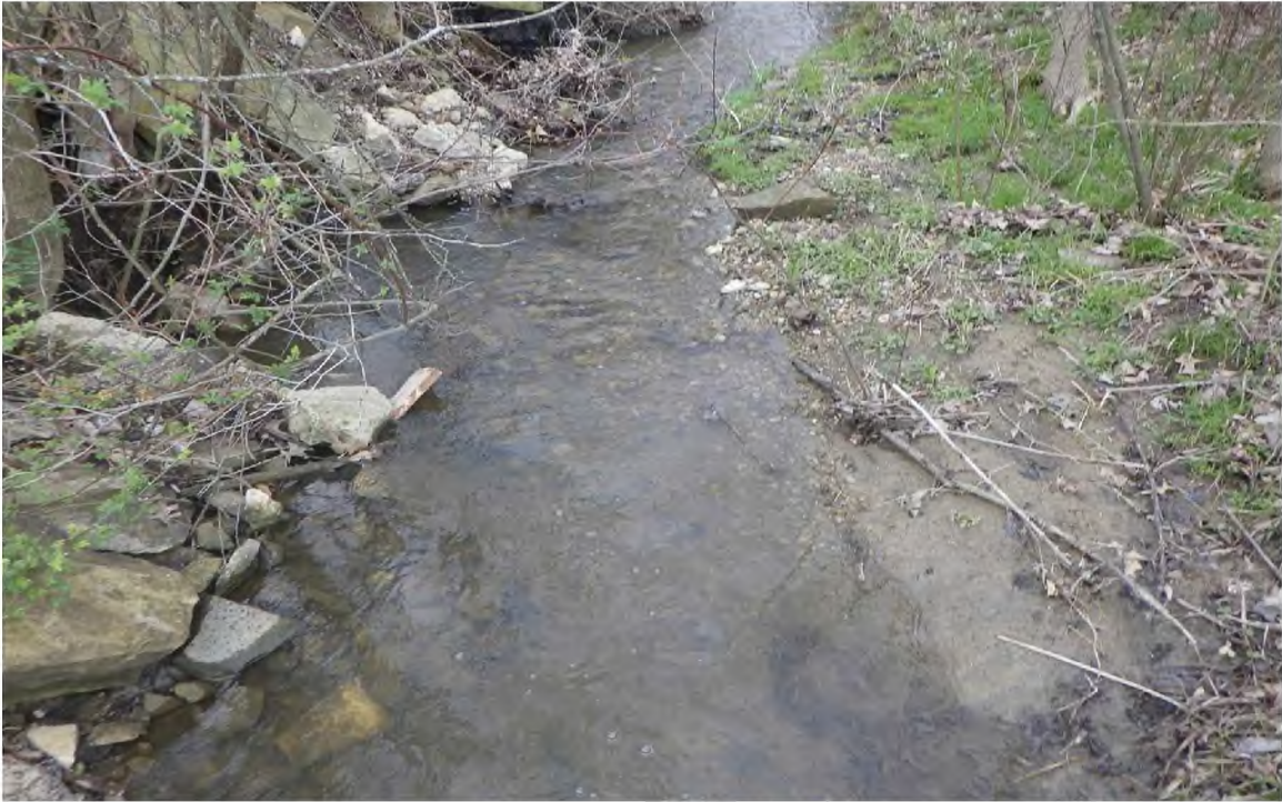
Photograph 95 View of Stream 1 (Blacklick Creek) substrate (west of Clover Valley Road). (EMH&T 4/19/22)
