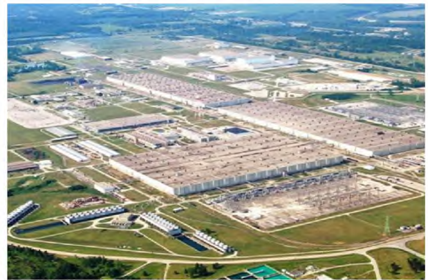
Portsmouth Gaseous Diffusion Plant
