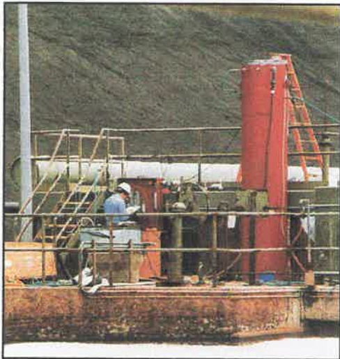
Full Depth Column Alpha Testing
