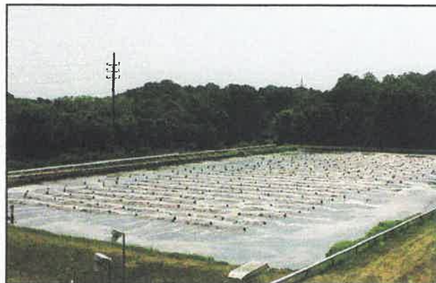
WETEC-TAS™ /AERGRID™ Retrofit Installation
