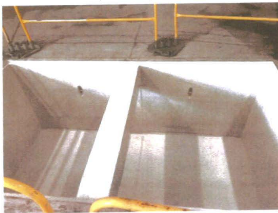
Sump after coating was applied.
