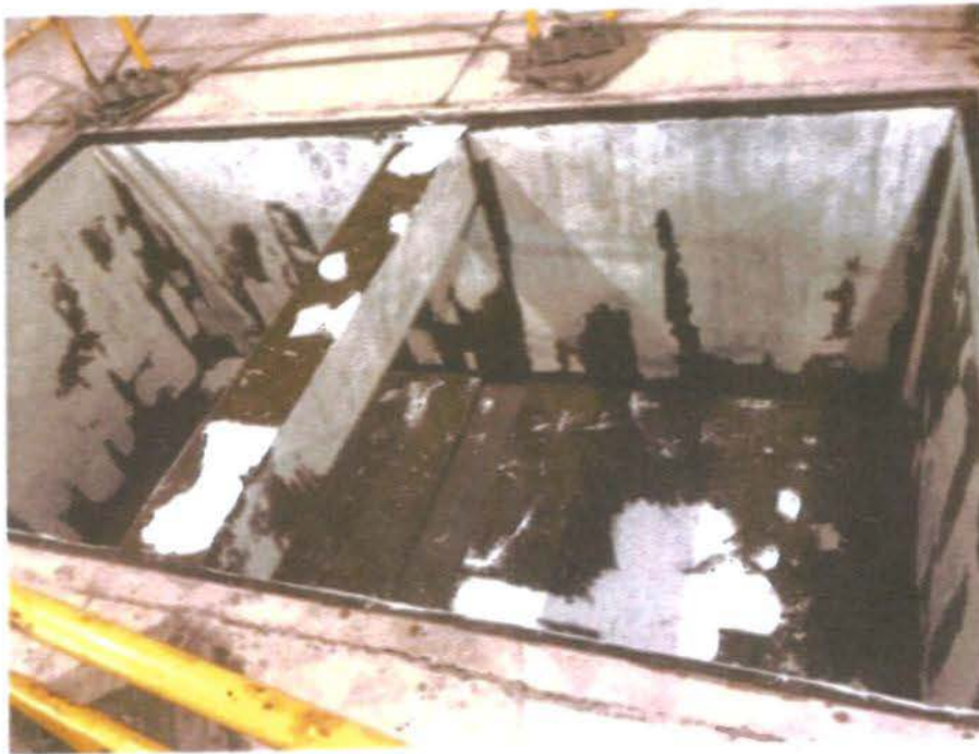
Sump during coating process.
