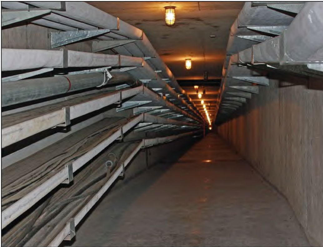
Figure 12. Typical Instrument Tunnel Prior to Deactivation
