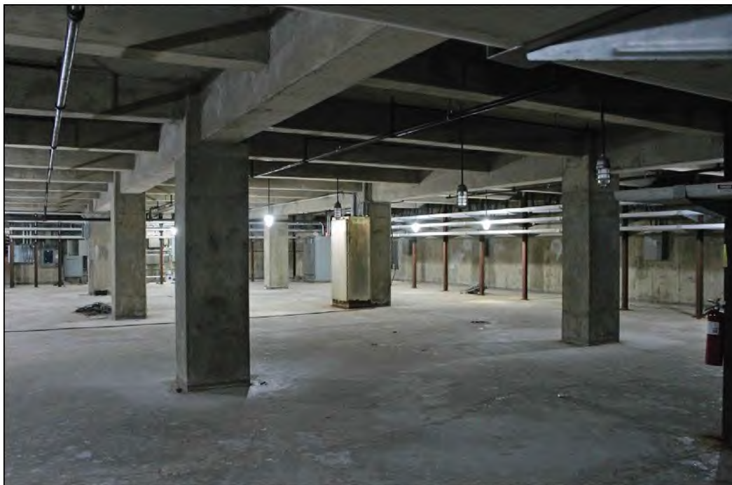
Figure 11. Typical Area Control Room Basement Prior to Filling with Grout
