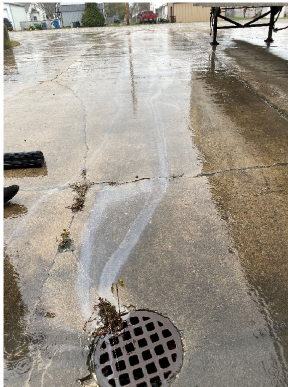
Figure 4. Sheen discharge into storm drain located in loading bay on west side of the facility.
