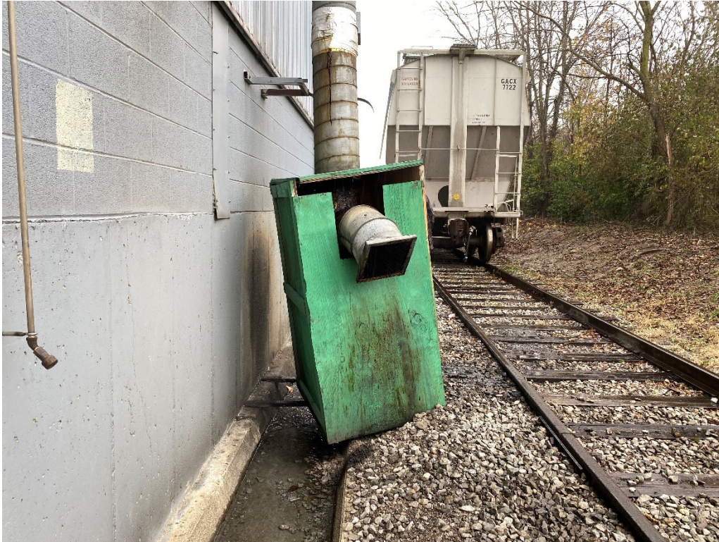
Figure 3. Air filtration particulate collection drum.
