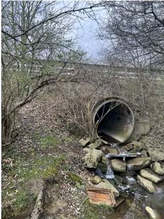
File Name: IMG_1118 DateTime: 2025:04:01 10:44:43 Latitude: 41.02989444 Longitude: -80.77777222 Description: Debris and rocks at base of culvert beneath the bike trail.
