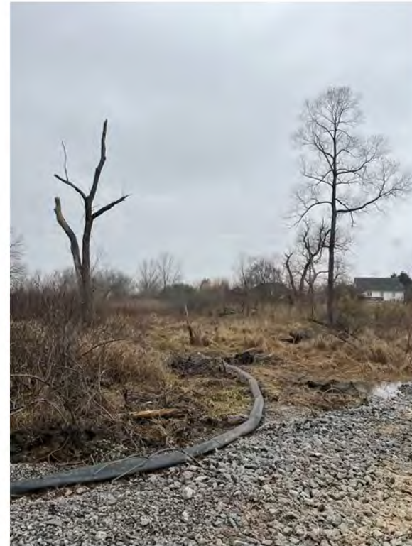
File Name: IMG_0588 Date/Time: 2024:11:21 14:13:20 Latitude: Longitude: Description: Temporary gravel access road, water bypass pump, wetland area.
