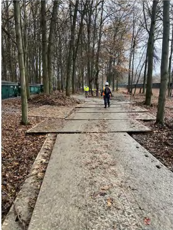
File Name: IMG_0584 Date/Time: 2024:11:21 14:08:16 Latitude: Longitude: Description: Temporary mud matting through upland forested area (ditch and temporary fencing along right side of photo).
