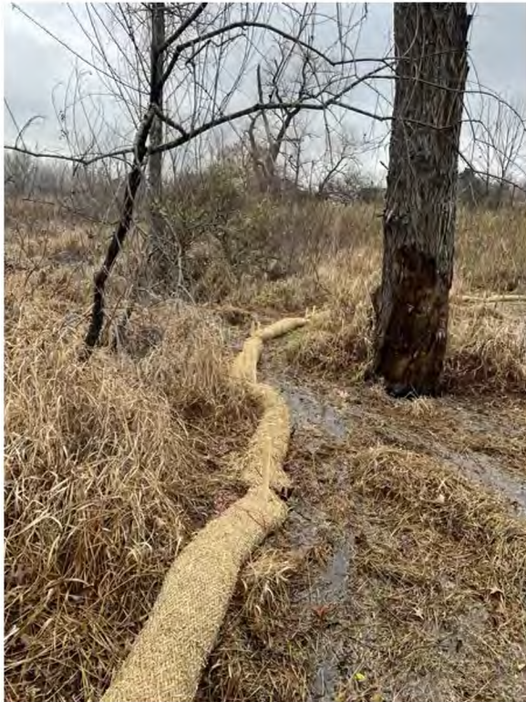
File Name: IMG_0711 Date/Time: 2024:11:21 15:34:31 Latitude: 41.02963889 Longitude: -80.77806111 Description: Sediment control measures around perimeter of standing water portion of wetland.
