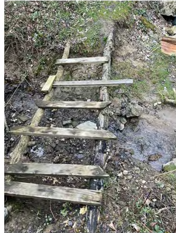
File Name: IMG_1117 DateTime: 2025:04:01 10:44:34 Latitude: 41.03011389 Longitude: -80.77787778 Description: Dilapidated wooden footbridge that crosses over the high school creek. Facing the culvert under the trail.
