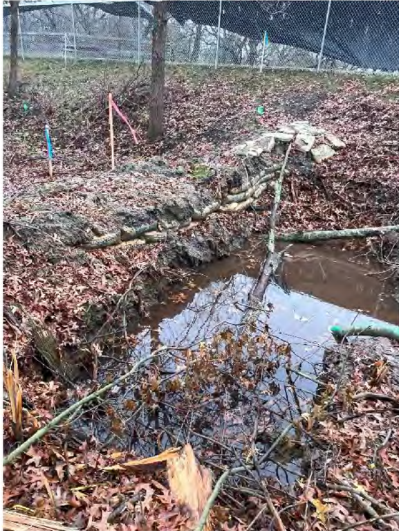
File Name: IMG_0599 Date/Time: 2024:11:21 14:20:32 Latitude: Longitude: Description: Temporary dam to collect water from Adjacent Ditch.
