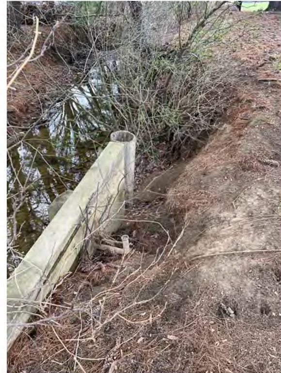
File Name: IMG_1166 DateTime: 2025:04:01 11:14:32 Latitude: 41.03063889 Longitude: -80.77628333 Description: Base of footbridge with erosion.
