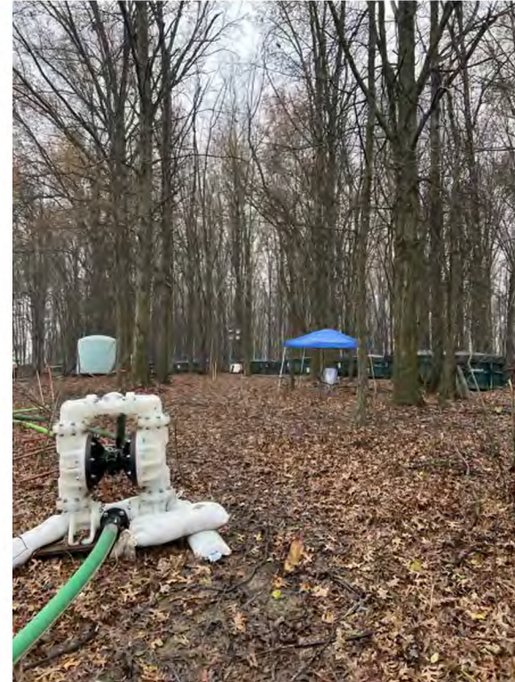
File Name: IMG_0604 Date/Time: 2024:11:21 14:23:00 Latitude: Longitude: Description: Bypass pump in foreground, roll off boxes staging area in background.
