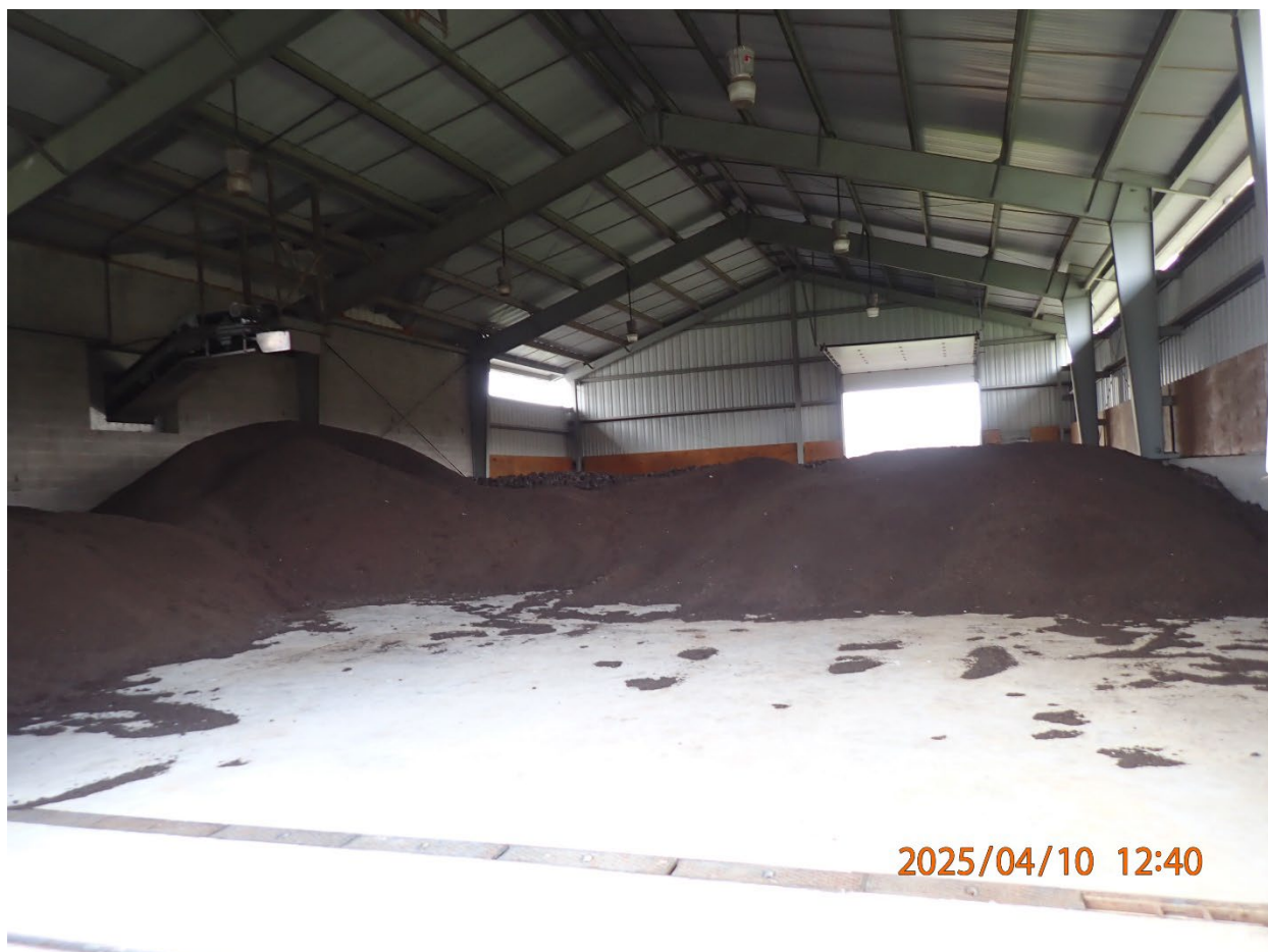
Figure 14. Biosolids storage pad. Photo taken 4/10/2025 by Whitney White. Pickaway Correctional Institution WWTP, NPDES #4PP00003.
