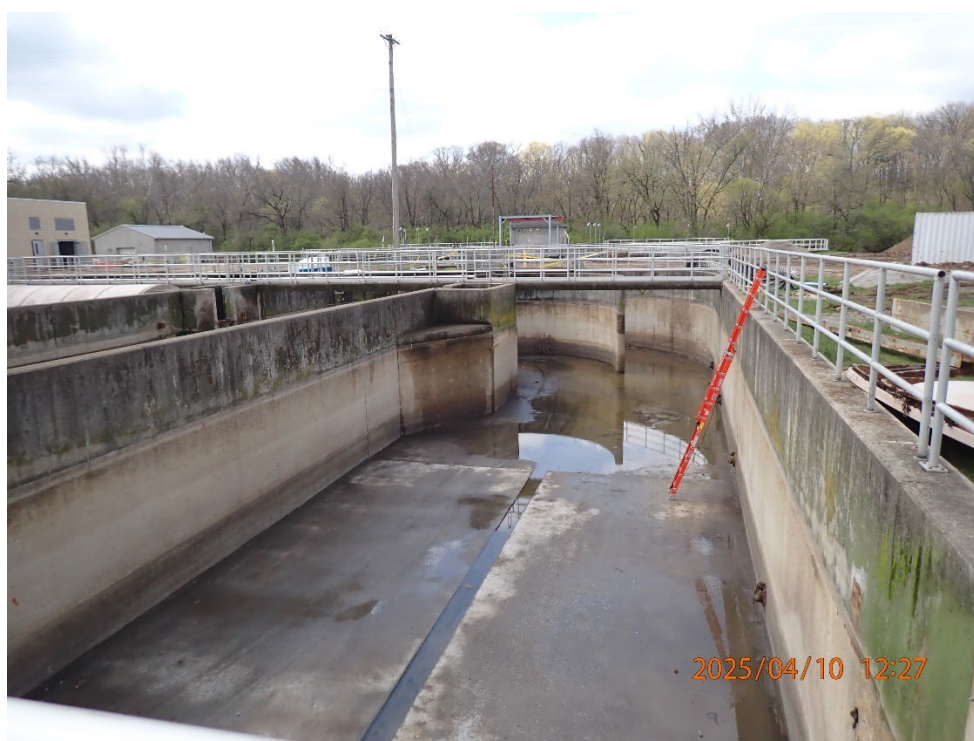
Figure 5. North oxidation ditch. Photo taken 4/10/2025 by Whitney White. Pickaway Correctional Institution WWTP, NPDES #4PP00003.
