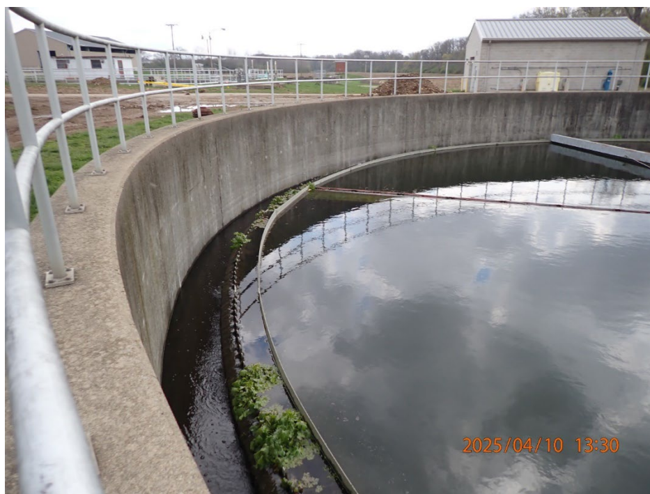
Figure 7. Clarifier Weir. Photo taken 4/10/2025 by Whitney White. Pickaway Correctional Institution WWTP, NPDES #4PP00003.
