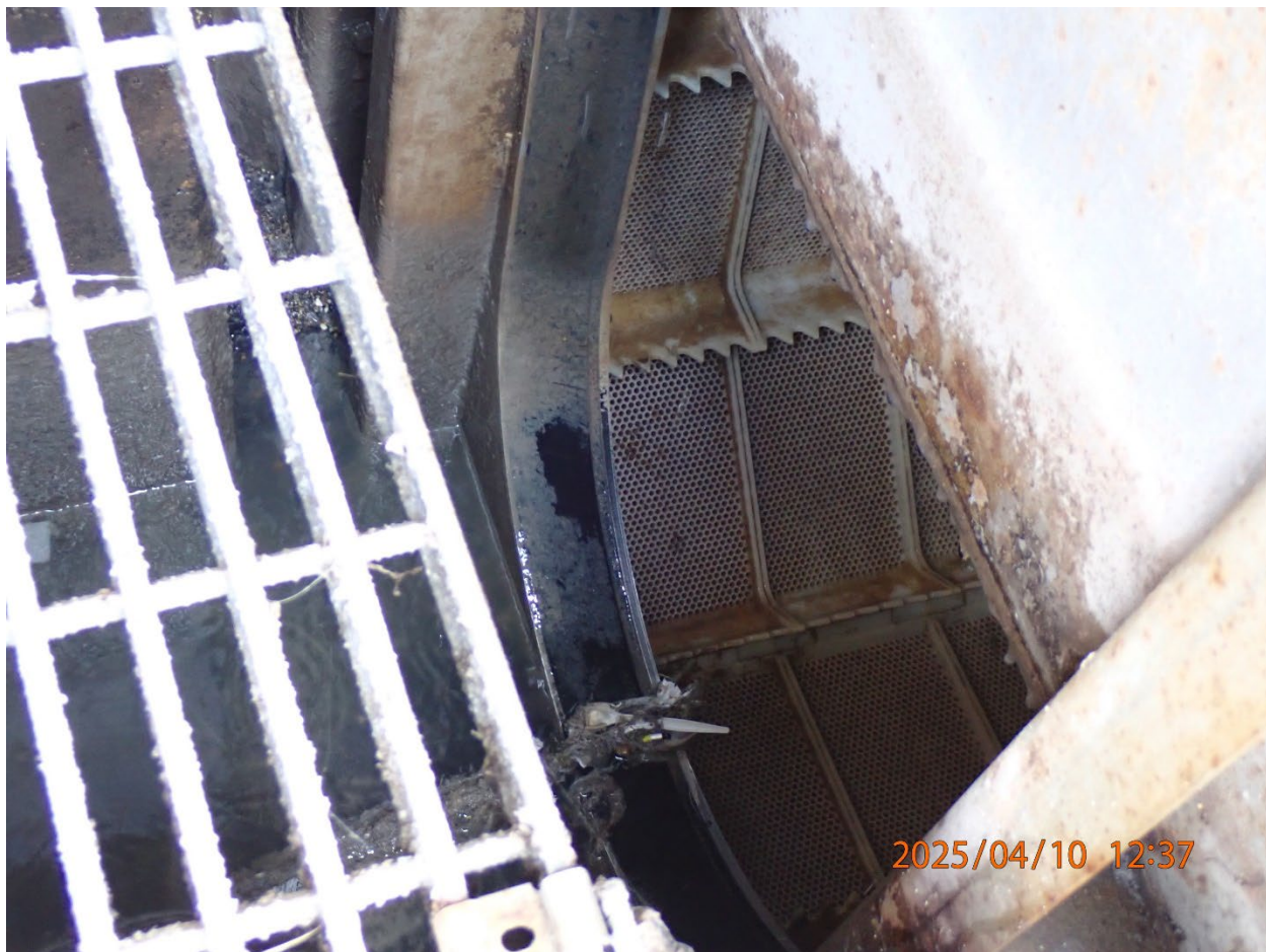
Figure 3. Band screen. Photo taken 4/10/2025 by Whitney White. Pickaway Correctional Institution WWTP, NPDES #4PP00003.
