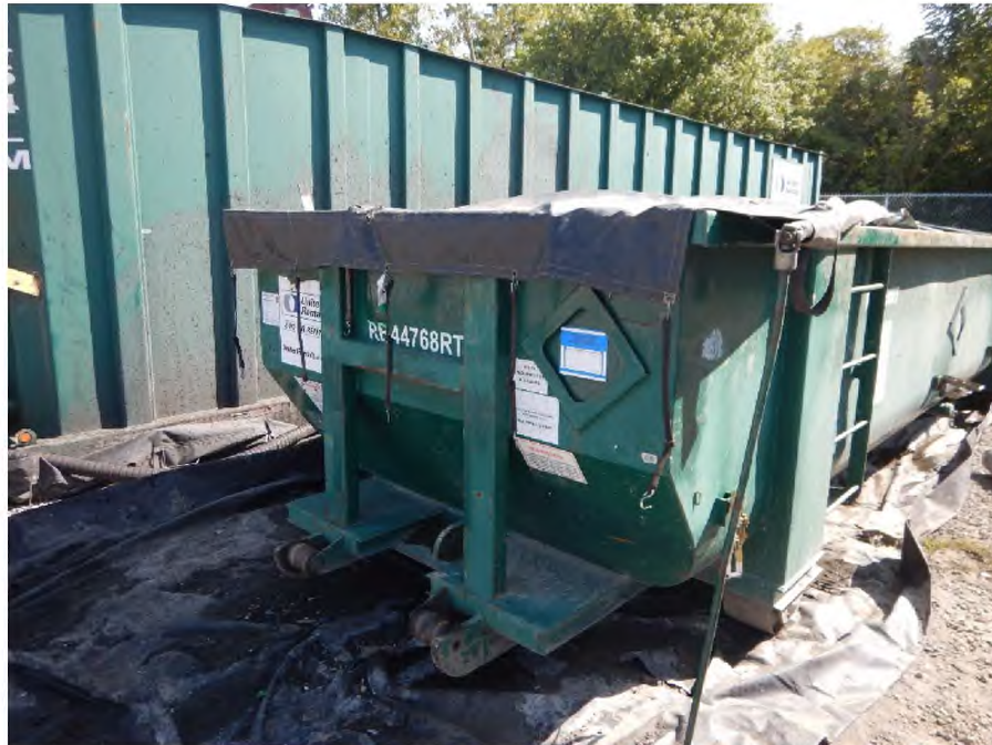
Photo 1 – Roll-off dumpster in eastern portion of gravel lot containing benzene wastewater and sludge (D018), unlabeled and partially uncovered at the time of inspection.
